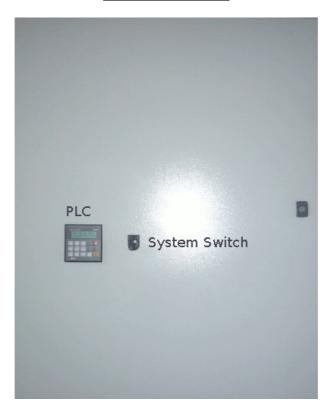
The control panel consists of a PLC controller, and a single system on off switch. On the next page is an image of the controller, with the relevant parts labeled by a white circle containing a number. Below the image is a key to the numbers giving the name of the item as it will be referred to in the rest of this manual.
